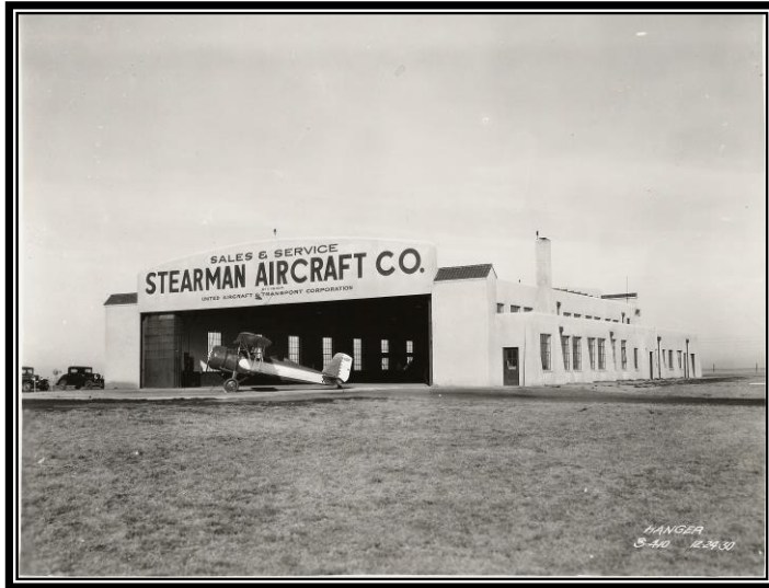
Figure 10. Stearman Hangar now known as Building 9 sometime in 1930 (Kansas Aviation Museum)
