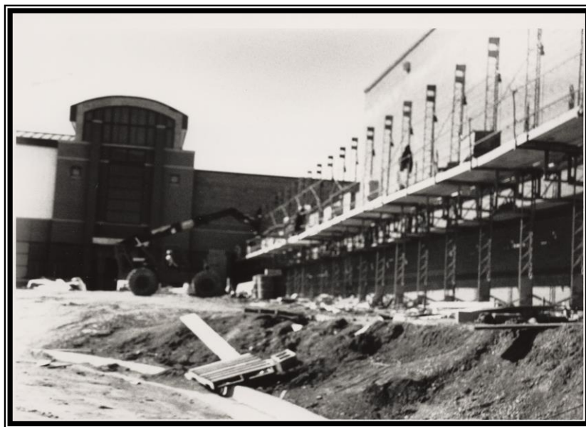
Figure 17. Emerald City (now the Robert J. Dole Community Center) under construction sometime in 1993.
