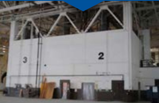
Building 1107, center support block for interior truss system (2010).
