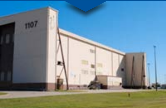
Building 1107, west side hangar door pockets, which contain the doors when they are fully open. These pockets are set beyond the walls so that the full length of the building can be opened when the doors are open (2010).
